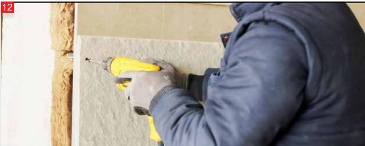
After fixing the laths, the next panel is brought over the strips and fixed in.
