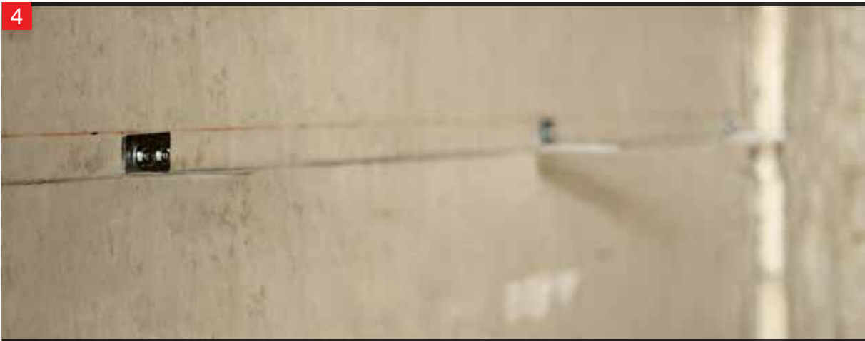
The L consoles for which the dowel locations have been marked are fixed into place using the right type of dowel.
