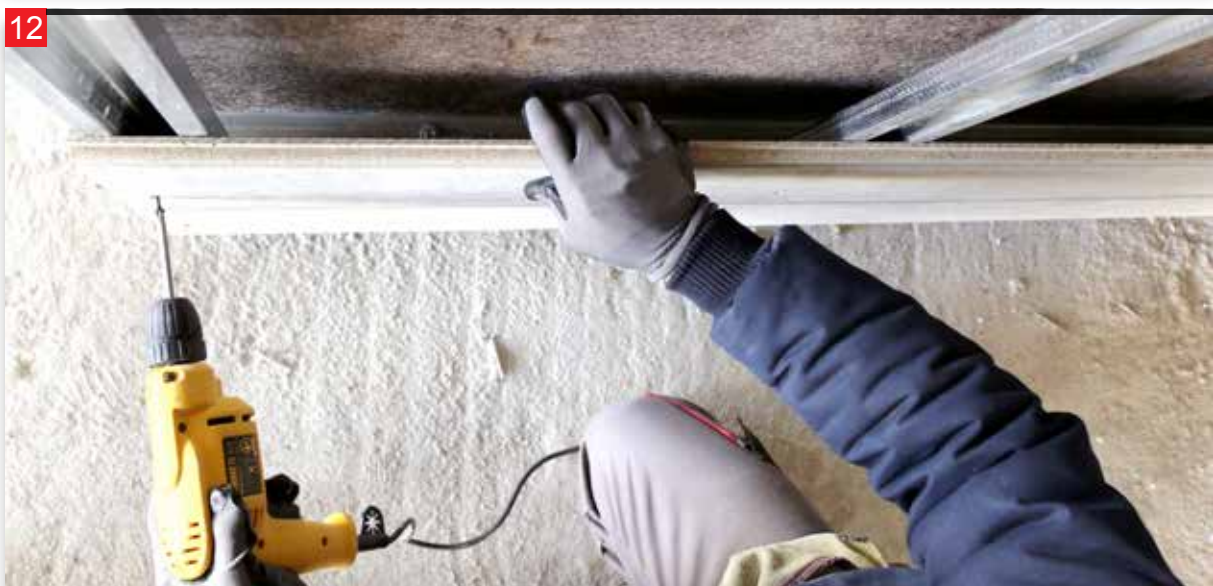
The aligned panels are screwed onto the M profile with anti rust screws.
