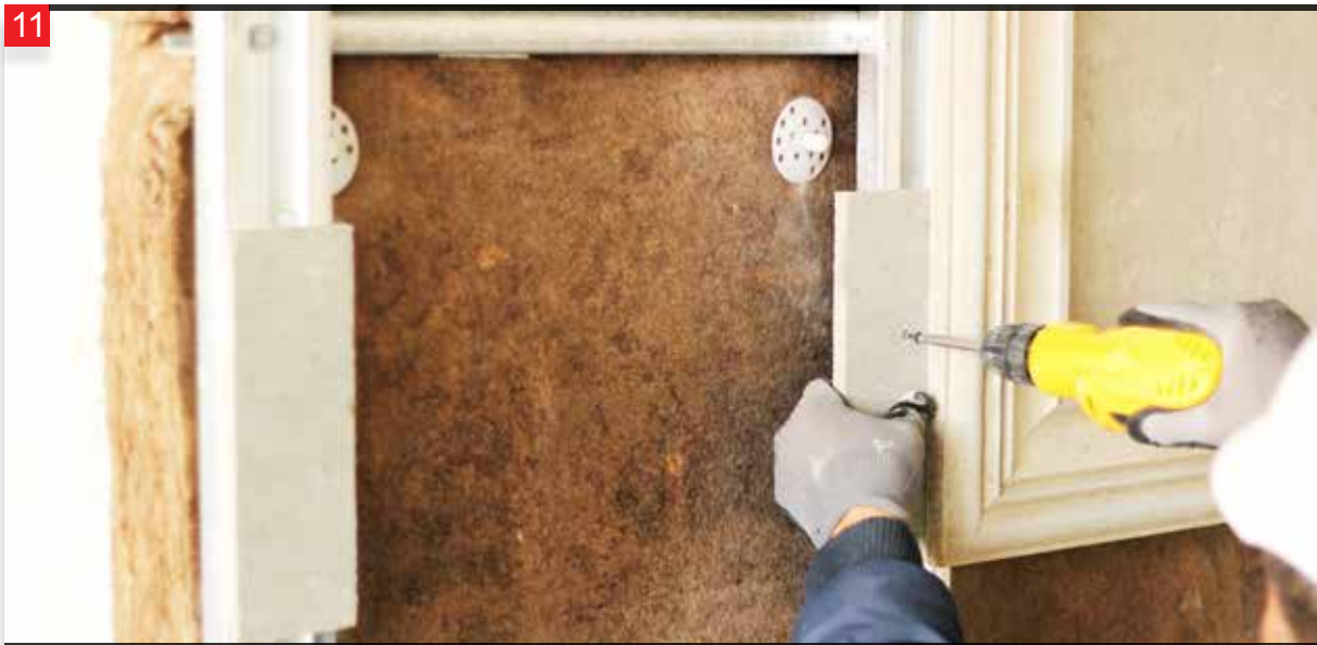
The strips are fixed on the M profiles so that the panel screw spots do not coincide.
