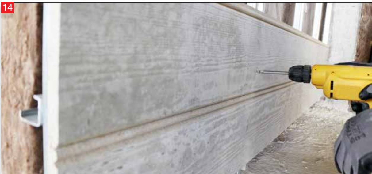
The screws are applied for each M profile and steps 5 through 14 are repeated for all the panels.
