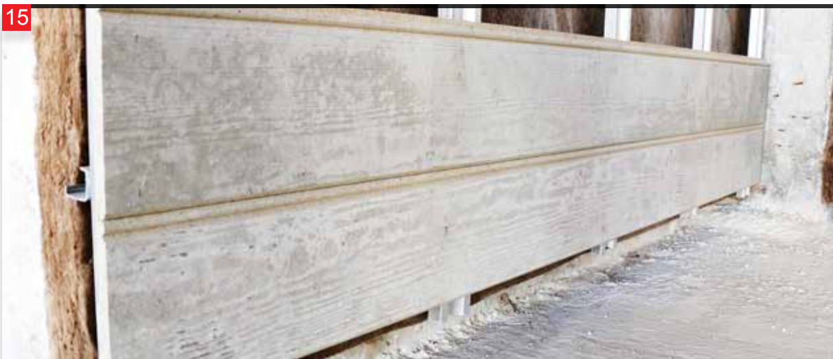
The screws are applied for each M profile and steps 5 through 14 are repeated for all the panels.
