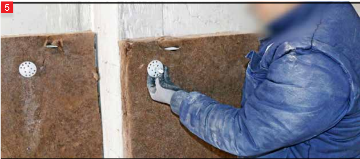
The desired thickness of insulation material is applied on the fixed L consoles.
