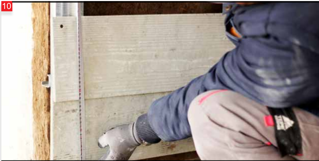
Measurements are taken for the subsequent panels.
