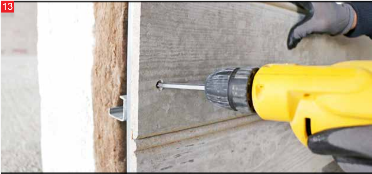
Carbon coated anti rust drywall screws should be used and driven in vertically.
