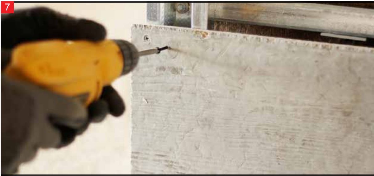
Screws are driven into the measured points as a guide to the overlap panel.
